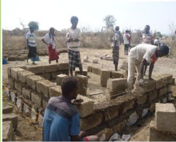
Working on Mud-block house construction - Awra
