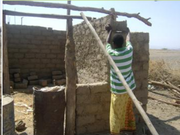
Working on Mud-block house construction - Awra
